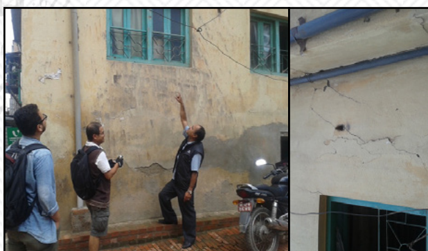
Engineers associated at EGBOSA carrying out Rapid Visual Damage Assessment for Ex-Gandakian
